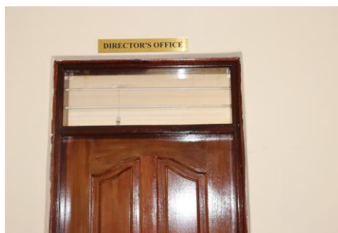
Even the doors are beginning to hint at what will go where.
